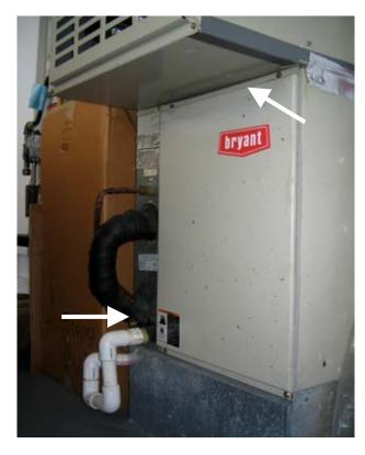
Significant air leakage was noted from the air conditioner box below the furnace in the garage. The seam between the box and the bottom of the furnace should be sealed and a threaded port at the bottom of the A/C box should be plugged to prevent excess energy loss.
