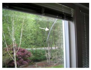
The lower level NW bedroom has one broken glass pane that should be replaced.
