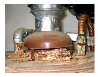
Heavy corrosion was noted on both water pipe connections on top of the water heater and around the flue. The water pipe connections were leaking at the time of the inspection. It is recommended that the pipe connections and the flue be further evaluated by a licensed plumber and corrections made, as needed.
