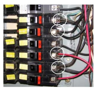
Double-and triple tapping (two or three circuits on the same circuit breaker) was found in the panel. Each circuit wire should be connected to its own breaker to avoid loosening of the wires at the breaker terminal. When the wires become loose, an electrical arc can occur, creating a potential fire hazard. Nuisance tripping due to overloading may also occur.
